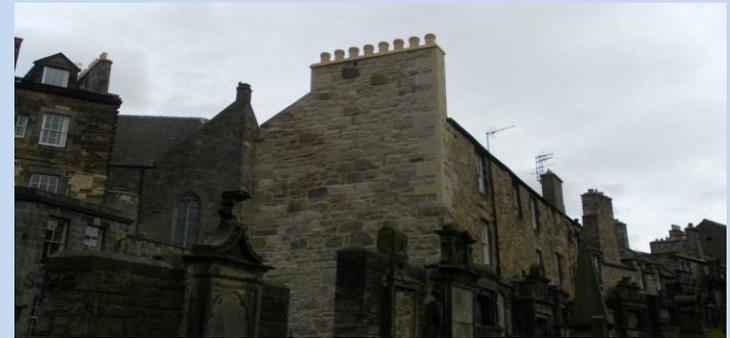
**Candlemakers Row** “has seen improvements to a category B listed building, which backs on to Greyfriar’s Kirkyard. Here a gable chimney stack had been repaired cheaply some years ago in brick and render, and the supporting stonework had begun to erode and crumble. The chimney has been re-built in stone, using buildings in nearby Merchant Street as an example”. (Quoted from *Edinburgh World Heritage*).
