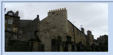
Candlemakers Row "has seen improvements to a category B listed building, which backs on to Greyfriar's Kirkyard. Here a gable chimney stack had been repaired cheaply some years ago in brick and render, and the supporting stonework had begun to erode and crumble. The chimney has been re-built in stone, using buildings in nearby Merchant Street as an example". (Quoted from Edinburgh World Heritage).
